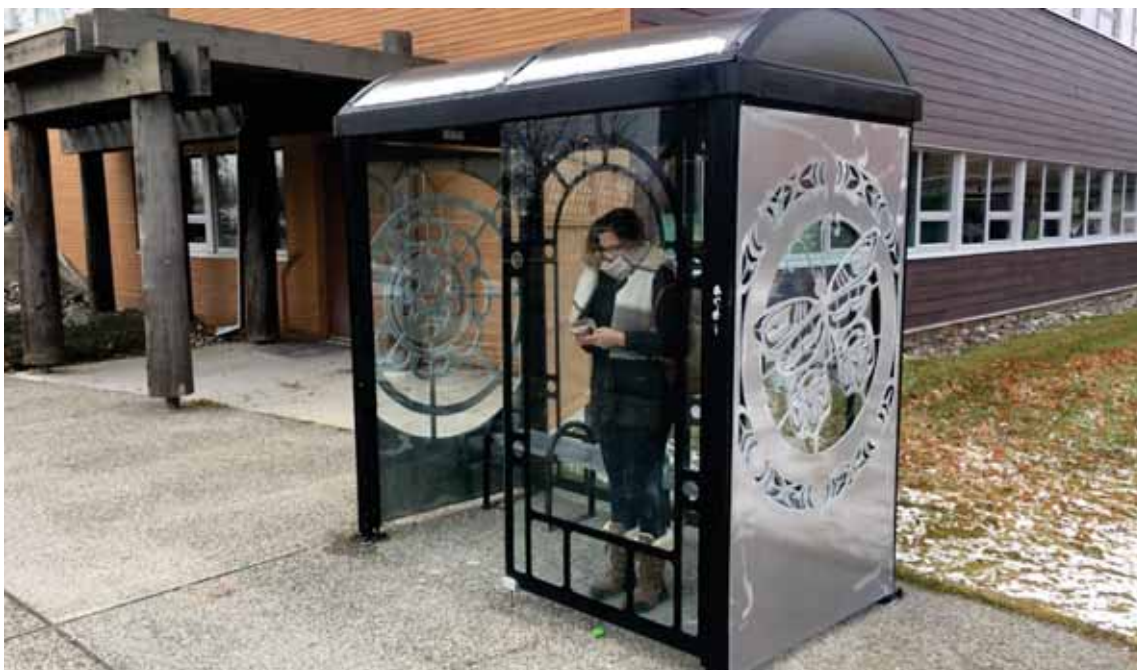
Figure 10: Current Whitehorse Transit Bus Shelter, Yukon College
