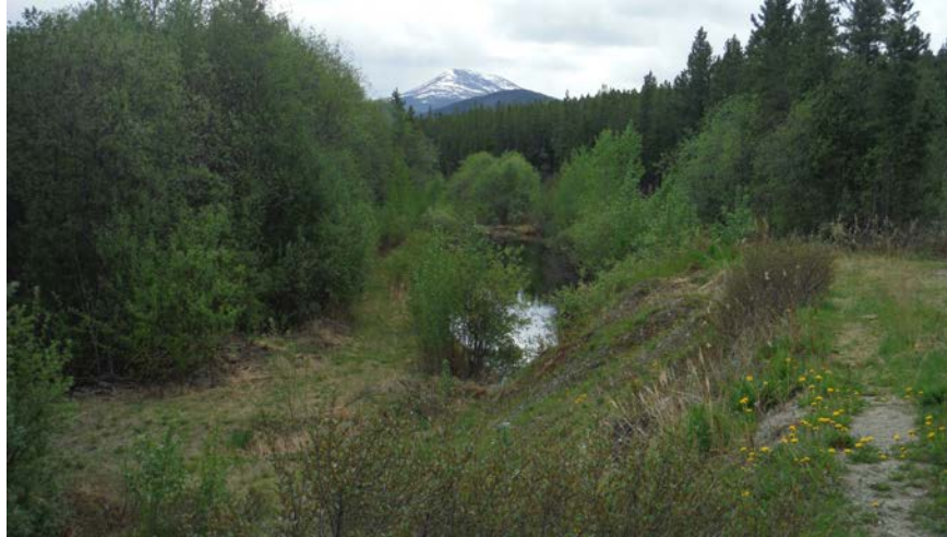
Figure 3: Small pond below third cell of Lobird sewage lagoons
