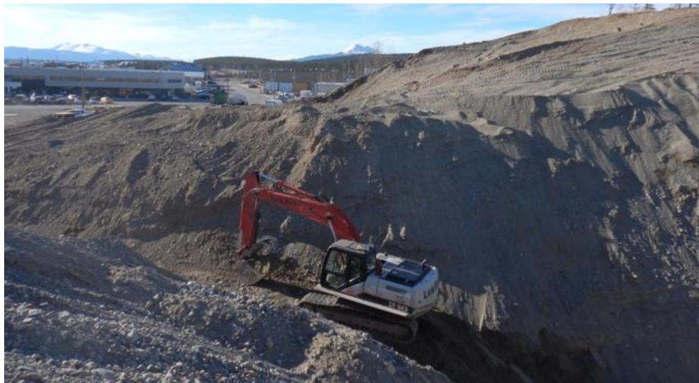
PHOTO 5. EXCAVATION TO REMOVE CONTAMINATED SOIL NEAR BURNS ROAD (GOLDER, 2019).
