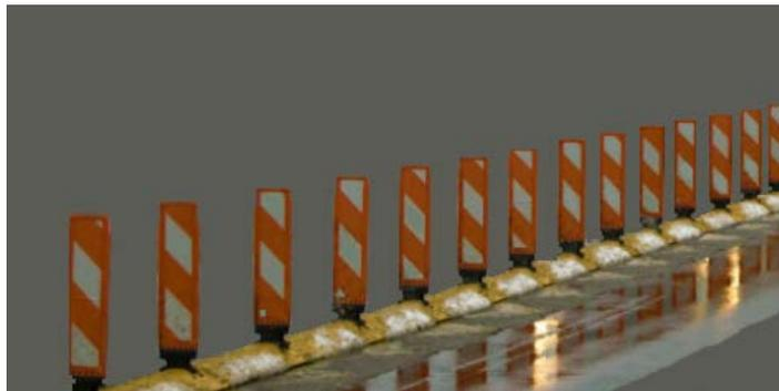
**Figure 4.12 B: Example of Curb-mounted Vertical Panels<sup>1</sup>**
