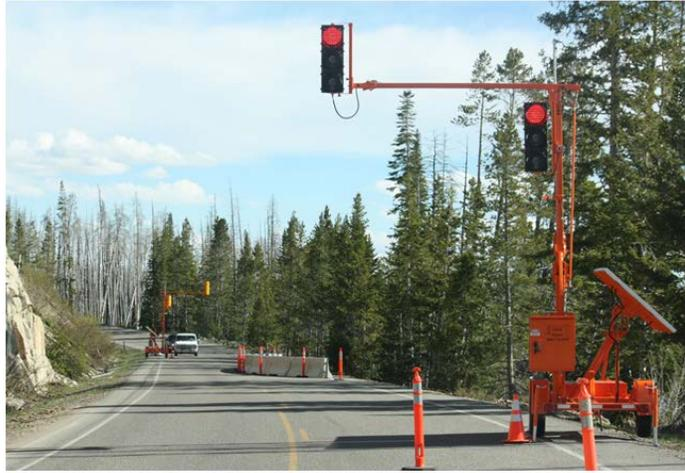
**Figure 4.22 A: Portable Traffic Signal Mounted on Trailer**
