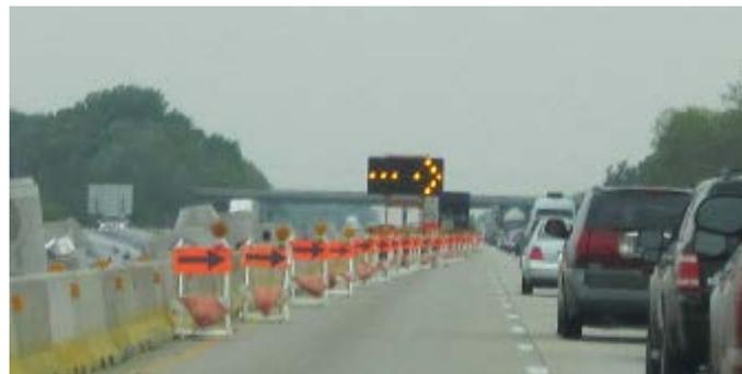
**Figure 4.13 B: Direction Indicator Barricade/Panels Used for Taper**
