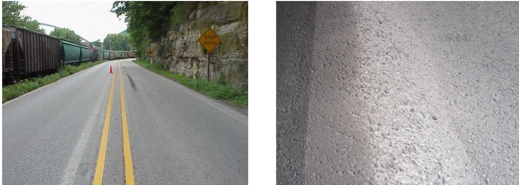
**Figure 4.2: Poor Eradication of Temporary Pavement Markings**
