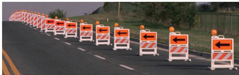
**Figure 4.13 C: Example of Direction Indicator Barricade/Panels used with Vertical Panels<sup>2</sup>**
