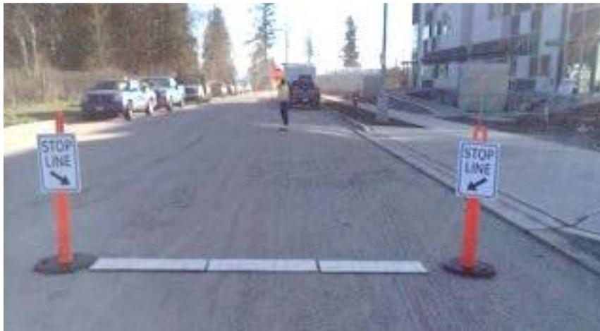
**Figure 5.8: Temporary Stop Bar**
