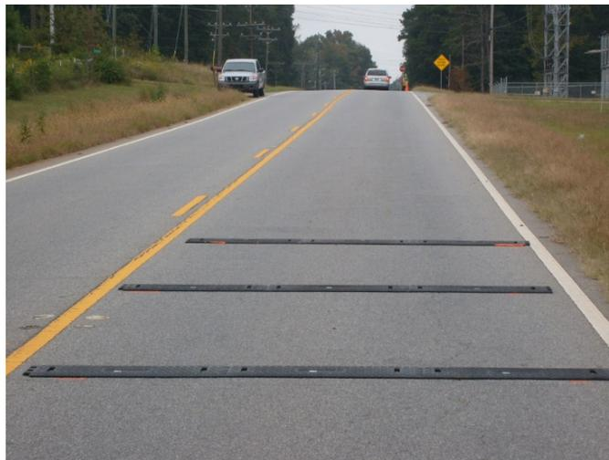
**Figure 4.30: Temporary Rumble Strips**
