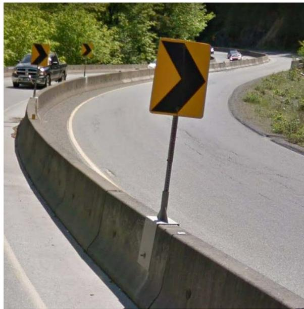
**Figure 4.1 B: Barrier Mounted Sign Supports – Saddle Brackets**
