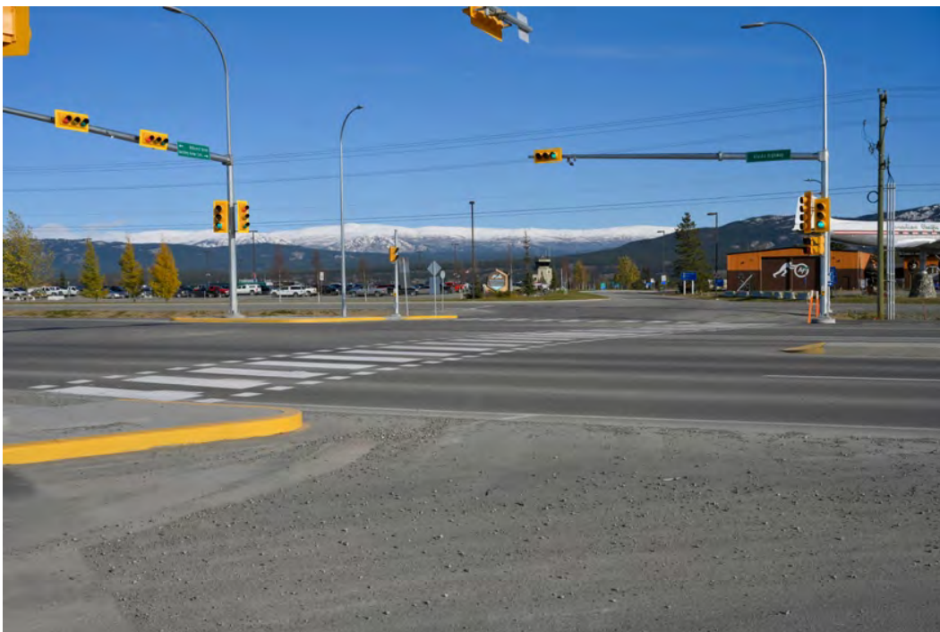
PHOTO 11: ALASKA HIGHWAY HILLCREST DRIVE BARKLEY-GROW CRES. SIGNALIZED INTERSECTION COMPLETED IN 2022
